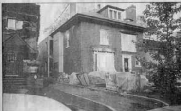
As the renovation got under way, (left), every window in the house was removed and several openings altered. Cast-iron radiators litter the back yard (middle) where a coach house
